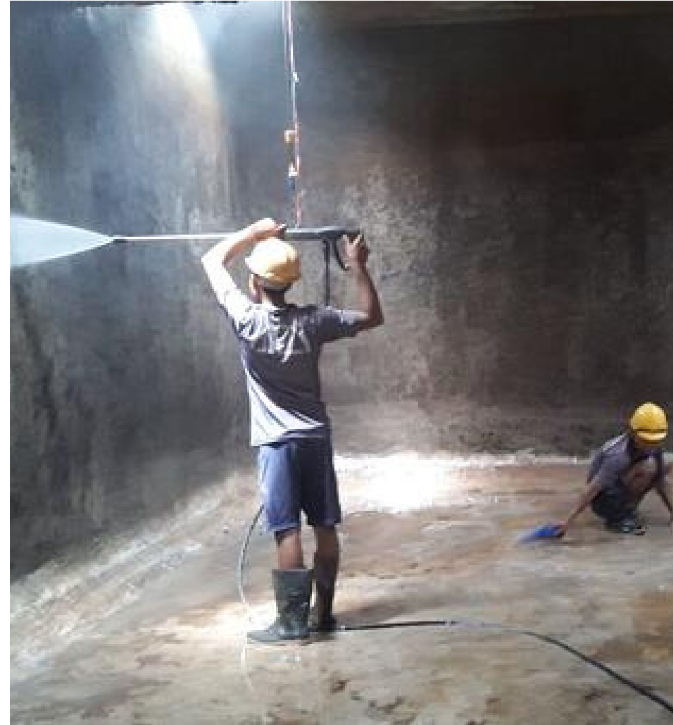
Building Water Tank Cleaning
